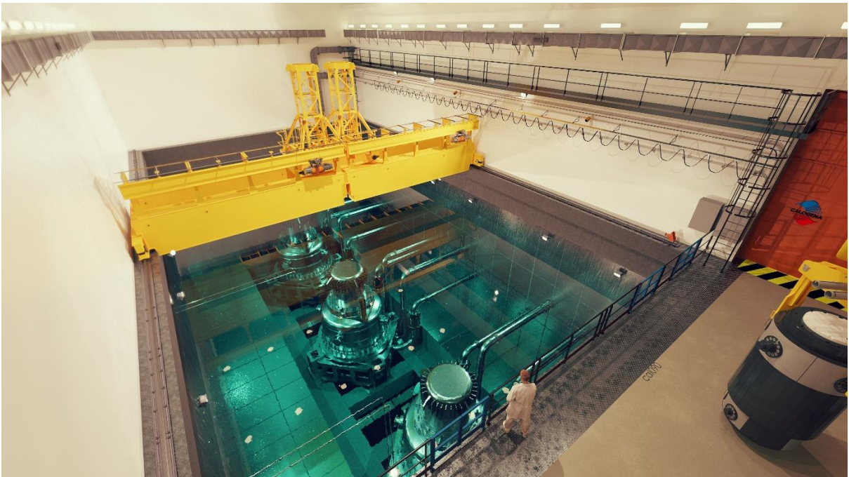
Internal view of a three boiler module
